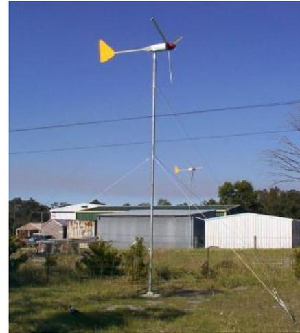
Figure 3: Guyed pole tower. Reproduced from <http://www.colgantoolmaking.com.au>
