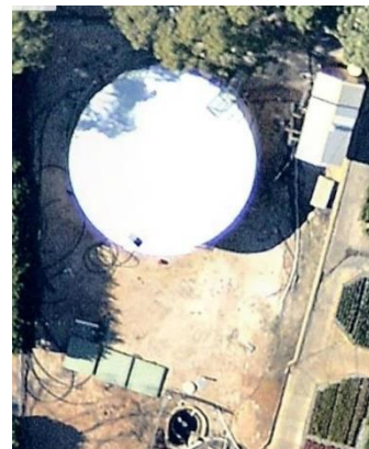
Figure 3 Domus Storage Tank 2017
